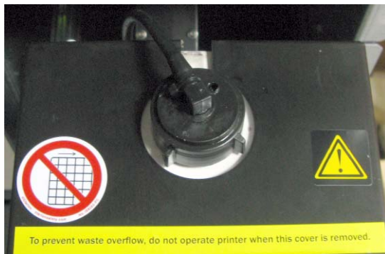
Figure 6-72: Fireproof cover installed over the waste container
